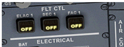
Picture 29 – Left FBW controls
