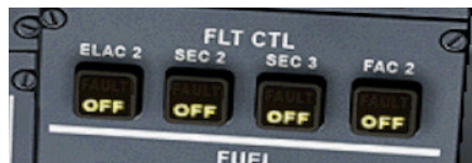
Picture 30 – right FBW controls
